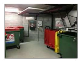
FireStop is a fully automatic 'water mist' fire suppression and protection system specifically designed for bin rooms in high-rise blocks.
